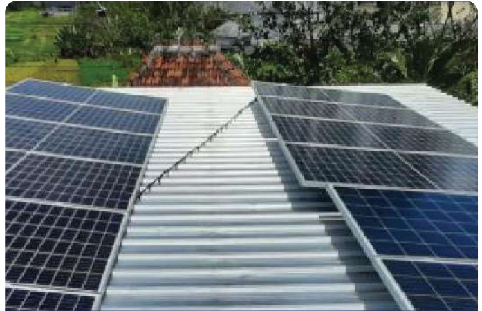
BALI SungaiWatch 4,67 kWp On-Grid System
